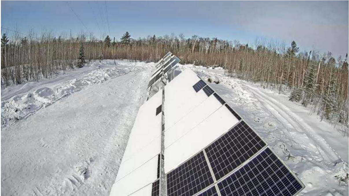
(b) Bifacial Modules at Dorval Lodge Completely Blanketed by Snow
