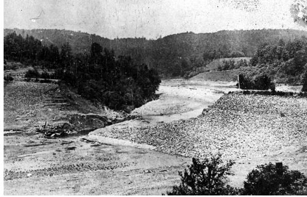
Figure I .9: South Fork Dam Failure in Wisconsin, USA (American Society of Civil Engineers, 1891)
