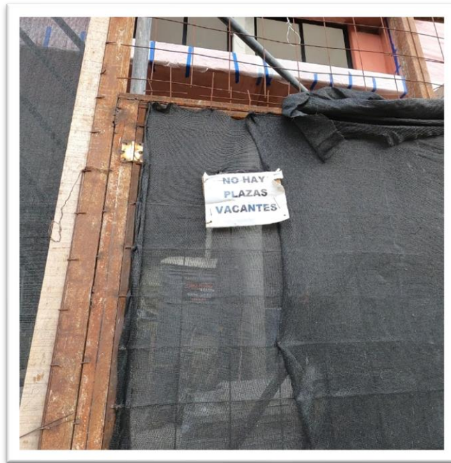
Construction site of Alma de Escalante building, 2019
