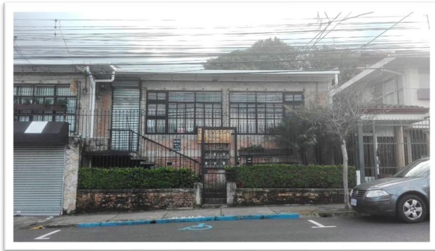
Image 249 Accessible parking, exclusionary buildings
