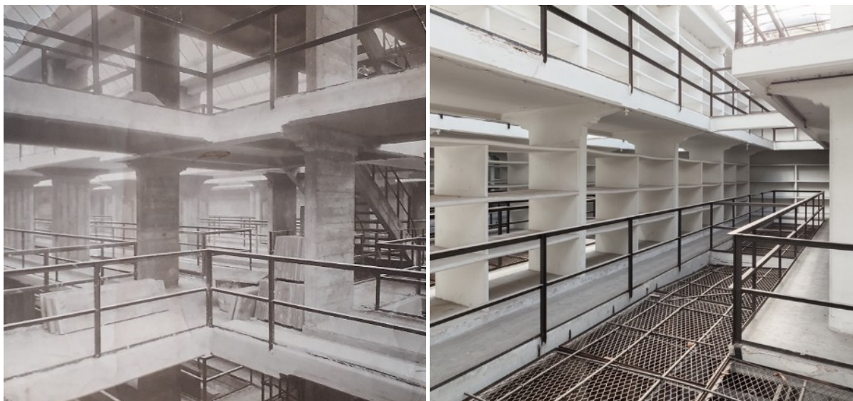
Figures 3.16 (a) and (b): The annex of Archives Départementales du Nord, Lille (Hainez, 1910) during construction, 1908-10 (left) and the building before reopening in 2022 after renovation (right), showing the extent of daylight admission via skylights as well as the béton armé system cantilevered balconies. (076 Ifa 108/10. CNAM/SIAF/Cité de l'architecture et du patrimoine/Archives d'architecture contemporaine & Nick von Behr)
