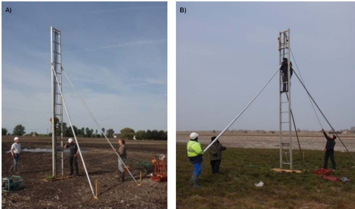
Figure 3.4. Pictures of core acquisition campaigns. A Bierne; B Les Attaques area.
