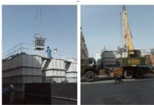
Figure 10: Membrane removal for external cleaning.
