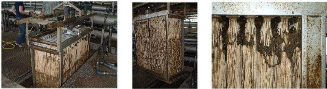
Figure 12: accumulation of sludge and hairs between fiber bundles due to faulty pre-treatment in the Hollow fiber membrane.
