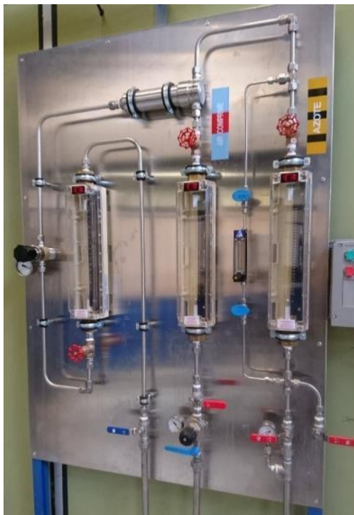
Figure 18: Air/Nitrogen regulation plate
