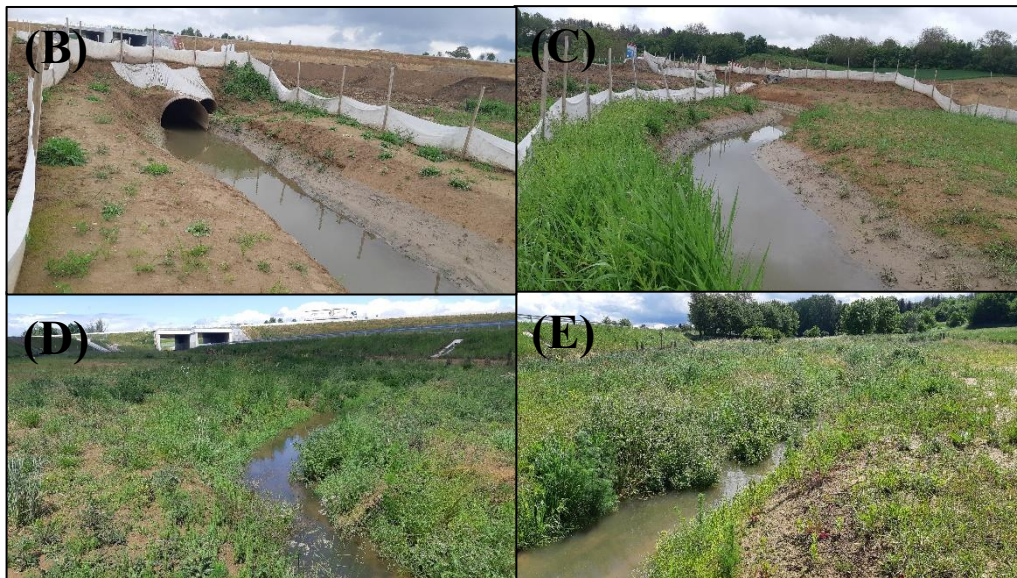
Figure S1: Historical monitoring of southern damselfly ( Coenagrion mercuriale ) populations and watercourse restorations 200m around the A355 (A); Photograph of a site sampled in 2021 (B, C) and 2022 (D, E). Watercourse drainage was visible in 2021 (B). Re-meandering work was carried out (C, E).
