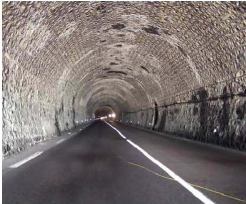
Figure 4.3. Photo of the tunnel where measurements were carried out.
