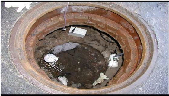
Installation of pH probe
