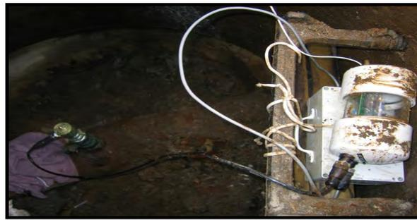
Installation of pressure sensor
