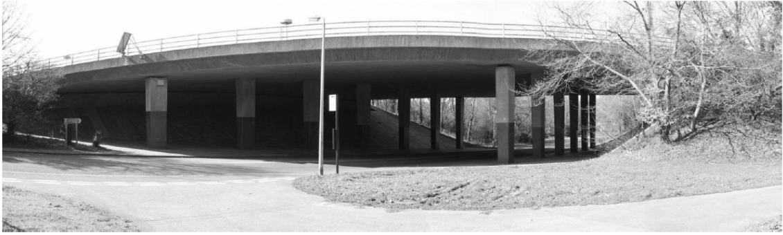
Figure 1.6: Pont du FerribyRoad [19].
