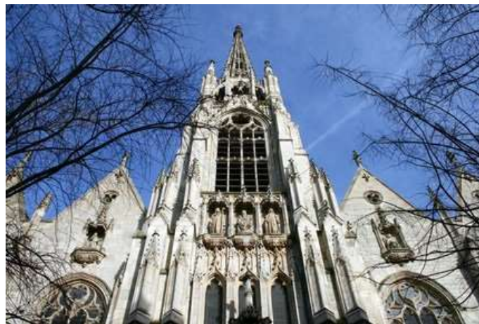
Figure 1.26. Cathedral of Saint Maurice in Lille constructed using the chalk extracted from underground layers.
