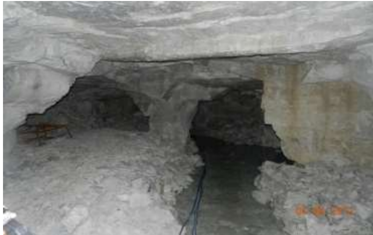
Figure 1.4. Rooms-and-pillars cavities in Hellemes, North France
