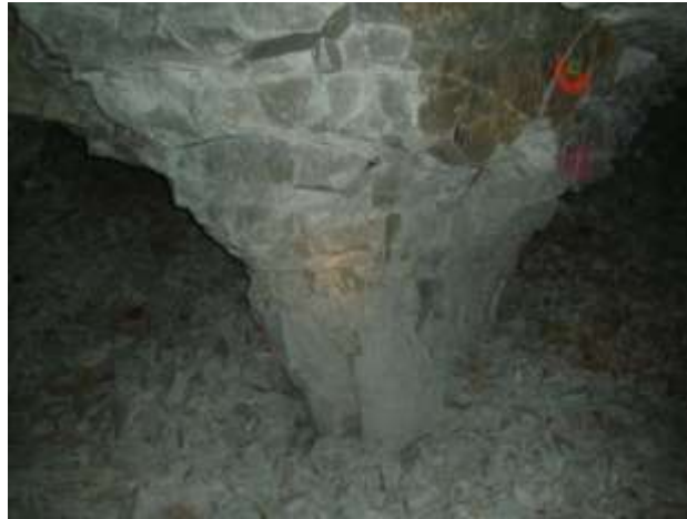
Figure 5.12. Pillar with reduced section from the cavity of Cavaignac, Lille.
