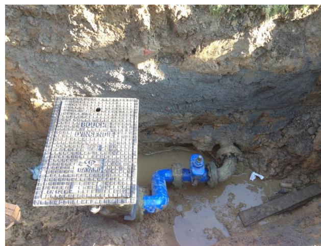
Figure 2.7: Hydrant before and after replacement
