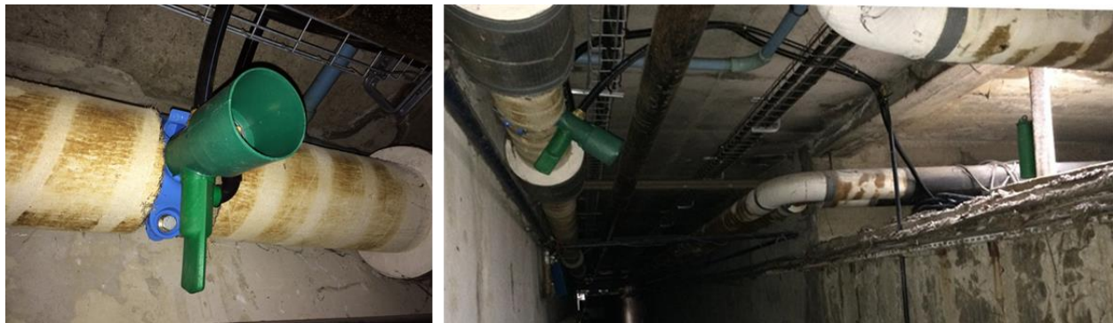
Figure 2.24: Installation of EAR system in the demo site
