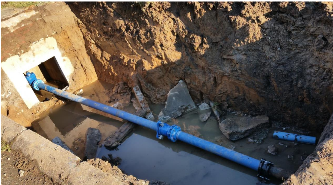
Figure 4.5: Leak repairs in front of the building M1
