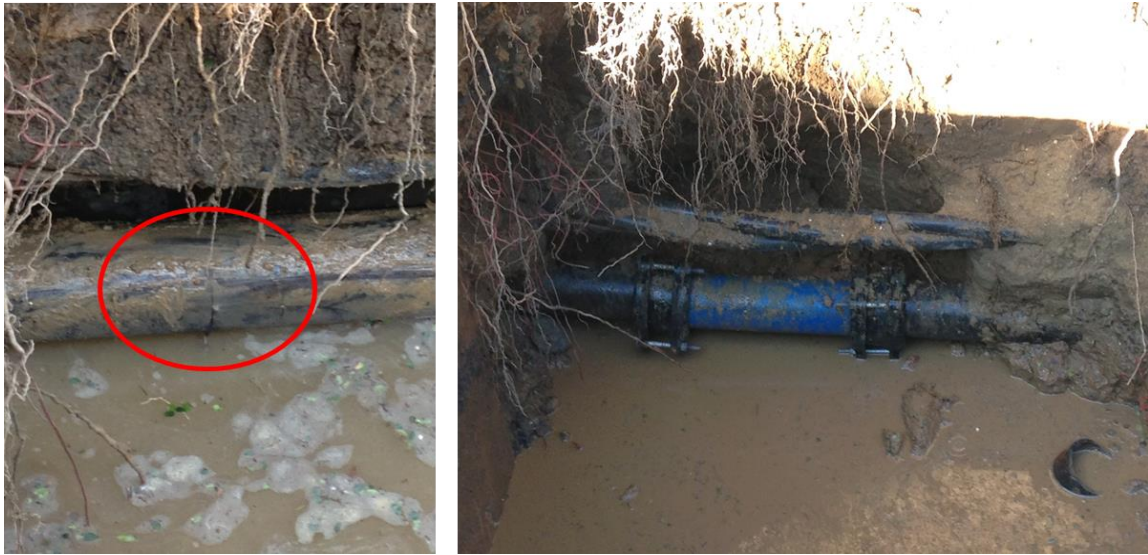
Figure 4.6: Leak repairs in front of the engineering school ECL
