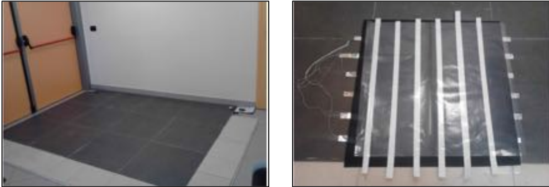
(a) The installed floor prototype
