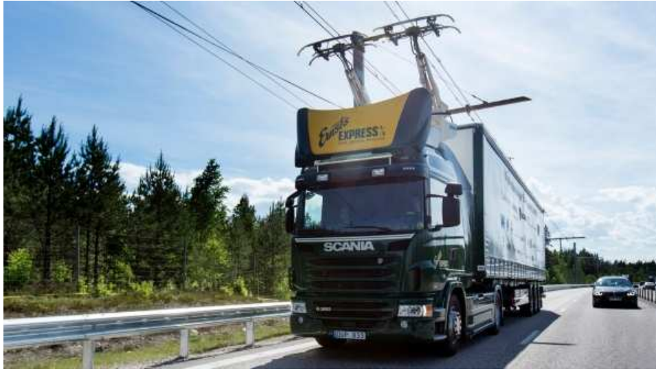
Figure 2.1 – Road freight transport powered by electricity [Sie17].
