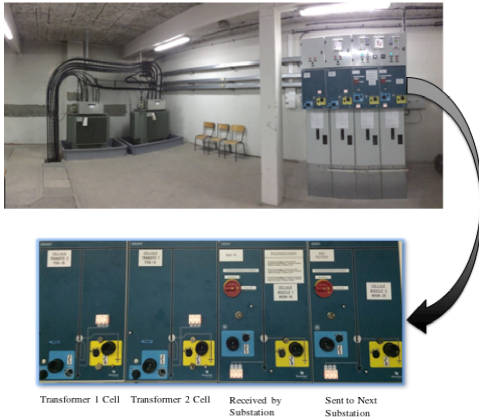
Figure 2.9 : The High Voltage component of the Substation
