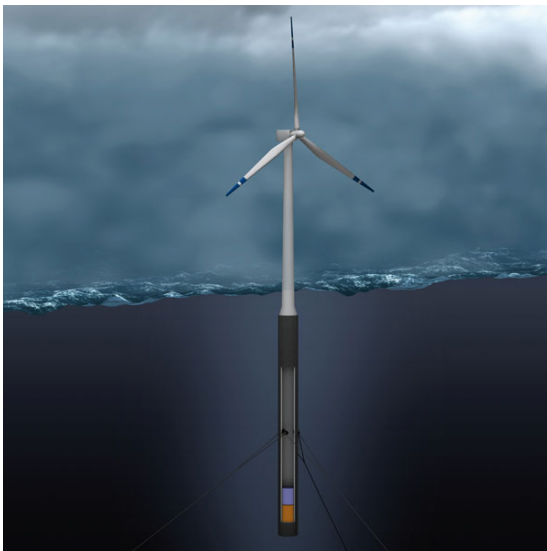
Figure 1.3 – Hywind 2.3 MW prototype deployed off the coast of Norway.
