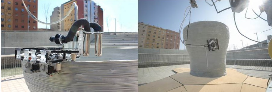
Figure 2.16 – IAAC Mini Builder from the University of Barcelona
