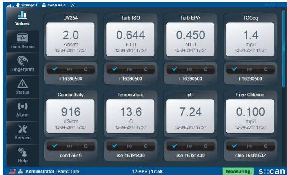
Figure 2.9. Example of data display from S::CAN sensor.
