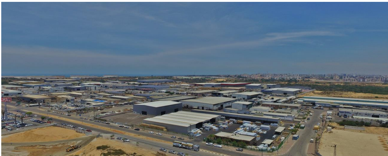
Figure 47: Industrial Buildings for Rental - Ashkelon Municipality.
