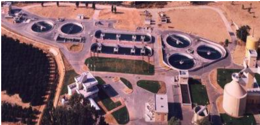
Figure 70: Waste Water Treatment- The secondary treatment is carried out in sedimentation basins, which contain large ventilators - Municipality of Ashkelon.
