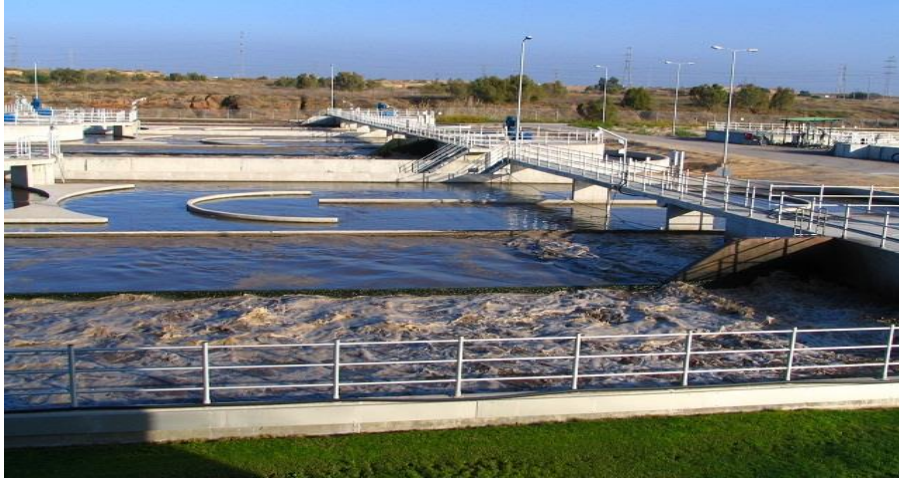
Figure 69: Waste Water Treatment- Primary treatment - Large bodies and sand in the raw sewage are removed - Municipality of Ashkelon.
