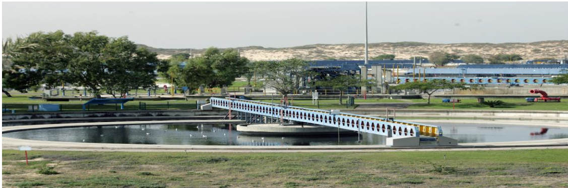
Figure 66: Wastewater treatment and effluent reuse - Mekorot Company website.
