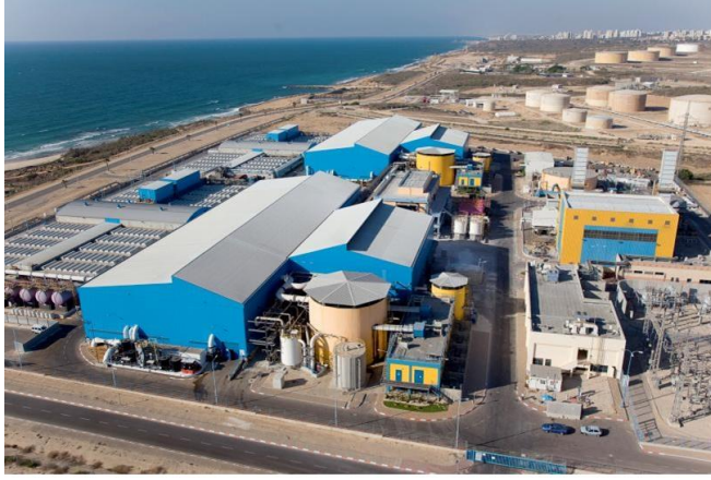
Figure 72: The Plant for the Desalination of Seawater in Ashkelon - Katsa Ashkelon company.
