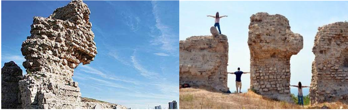
Figure 7. Byzantin wall years 324-638. Ashkelon municipality.
