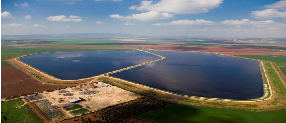
Figure 68: Stormwater Catchment – Mekorot Company website
