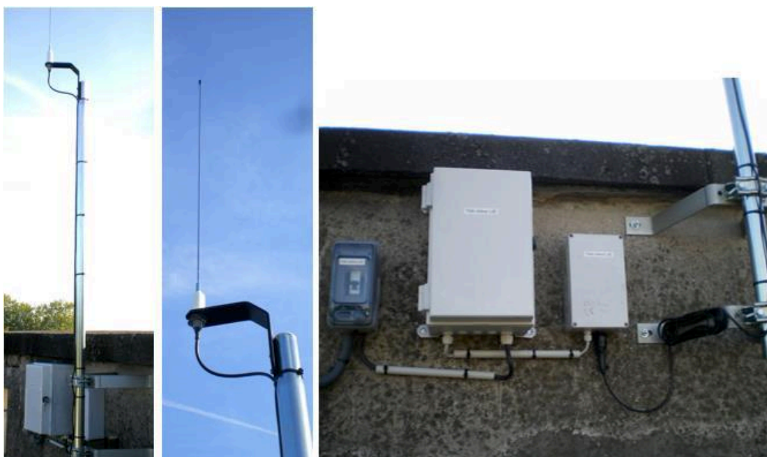
Figure 2.12 Data collector - Water distribution system of the campus
