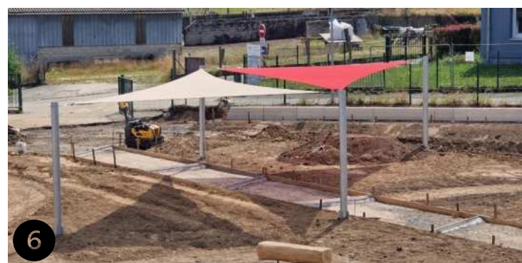
Figure 62 - Photo installation toiles tendues, cour Blangy-sur-Brelse ©P. Leroy, 2025
