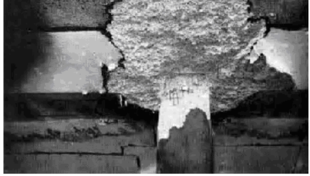
Port of San Francisco, piles 27&29
