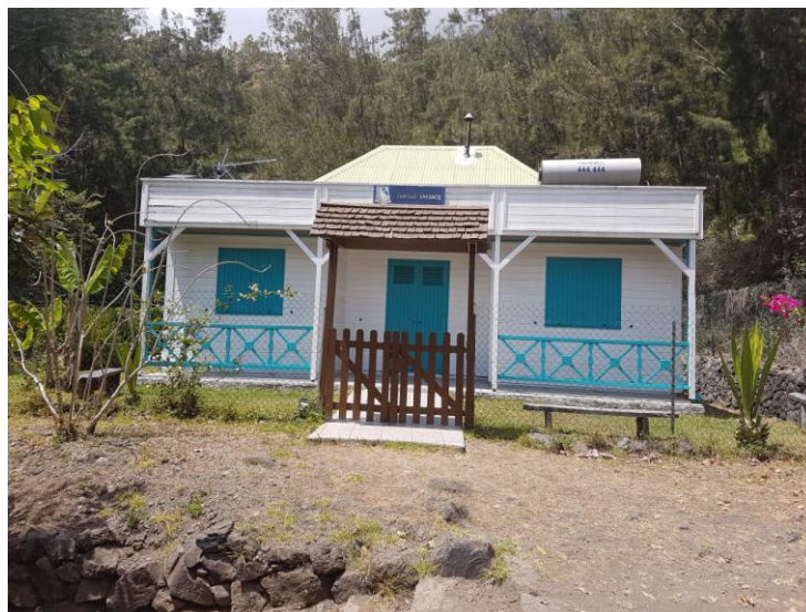
Figure 23: PMI de Roche plate (Photo KONAREFF P.)
